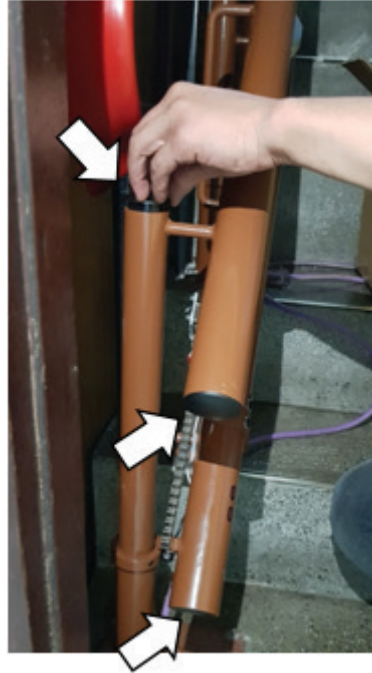
Figure 2.7 Tube Plug Locations
