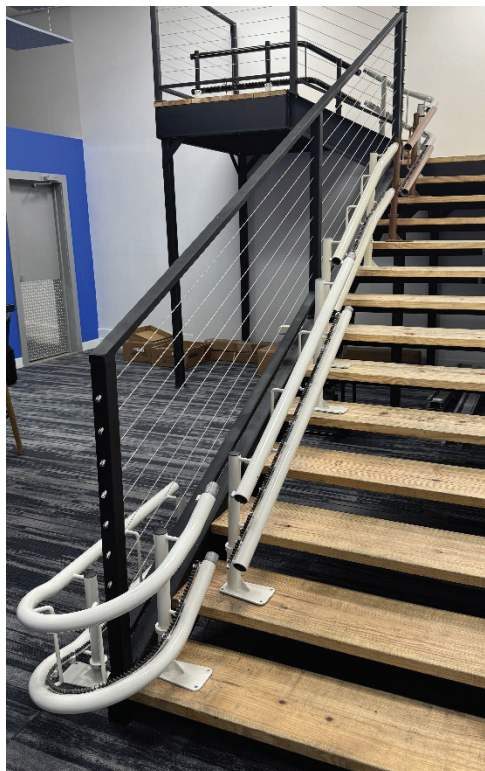
Figure 2-2.1 Staging of Rail Sections
