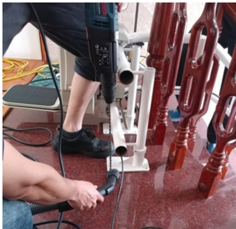
Figure 2.4.2.1 Concrete or Marble install Figure 2.4.2.2 Wooden Staircase install
