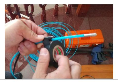
b.) Insert the Wire Threader with the Wire Harness from the topmost Rail Section through the Lower Rail of each Rail Section. Please Insert the Wire Harness through each Rail Section and Pull it to the adequate length. Repeat these actions until the Wire Harness is pulled out from the lowest Rail Section.
