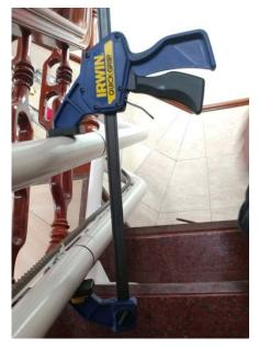
c.) Tighten the 1<sup>st</sup> and 2<sup>nd</sup> Rail Section by using an M6x35mm Screw. Make sure this screw is tightened from the upper end to the lower end of the Rail Joint.
