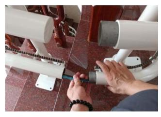
[Note] Make sure to adjust the length of the Wire Harness after putting it through each Rail Section instead of several Rail Sections. It will be too heavy to pull after it passing through 2 or more Rail Sections.
